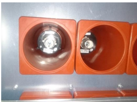
Sensors mounted on CB static contacts
