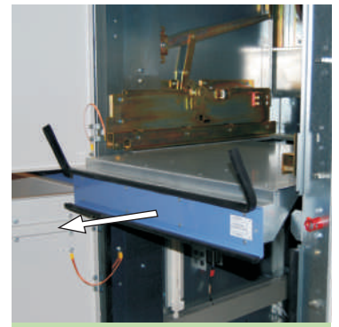
Removing partition between draw-out element and cable compartments
