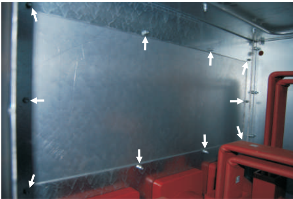
Removable access panel to busbars in circuit breaker compartment
