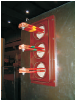
Busbar with special cast resin bushings
