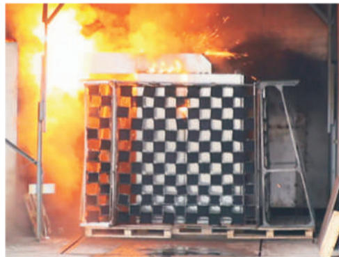
Internal arc test at 25kA/1s
