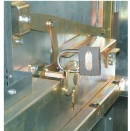
Locking shutter operating mechanism
