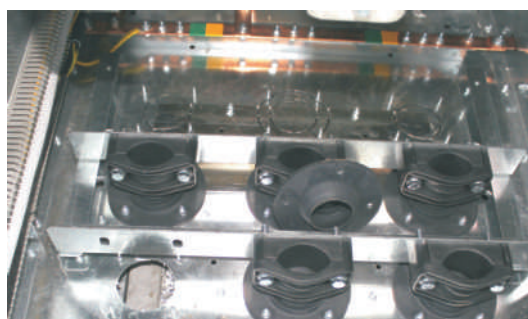
Bottom of cubicle hermetically sealed with cable entry sealing inserts
