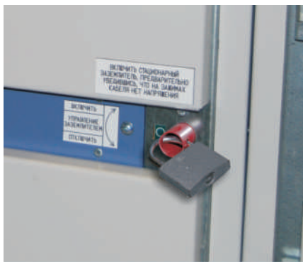
Locking earthing switch mechanism
