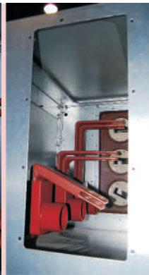
Removable access panel to busbars in circuit breaker compartment
