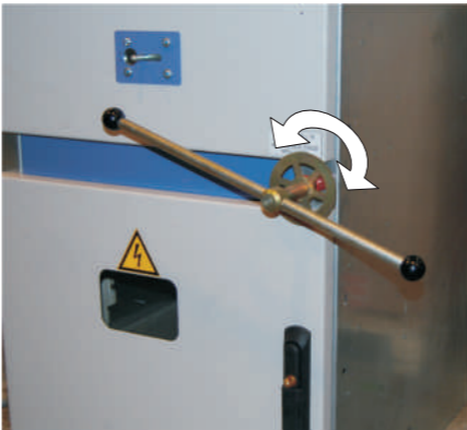
Handling earthing switch
