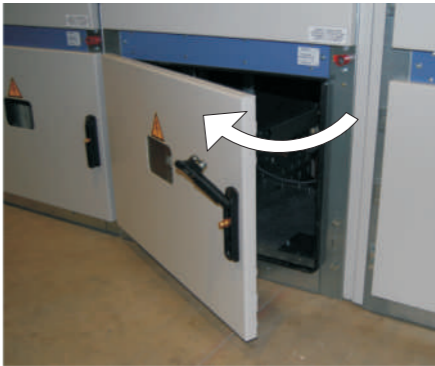
Opening cable compartment door
