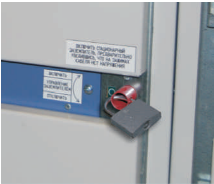
Locking earthing switch mechanism
