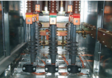
Fixing the cables and connecting cable earthing braid
