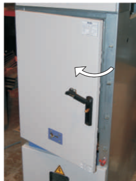
Opening draw-out element compartment door
