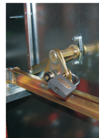
Locking shutter operating mechanism
