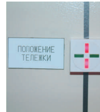
Electronic indicator of draw-out element status
