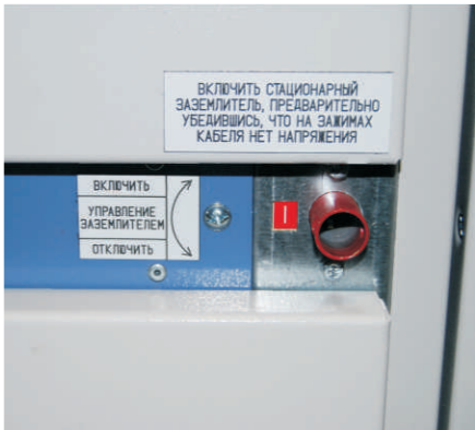
Mechanical indicator of earthing switch status
